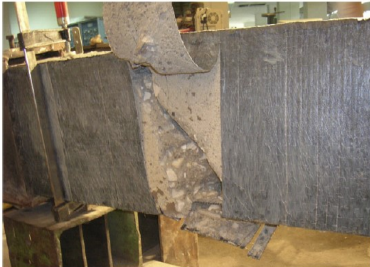
Fig. 6. Crack pattern of the fully and completely wrapped rectangular beam Rb-F(1) with continuous FRP sheets (FRP sheets partially removed).
