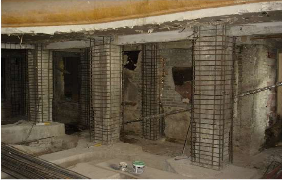
(c) Jacketing of the ground floor columns
