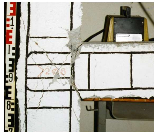
a. Initial loading ( failure mode-A )
