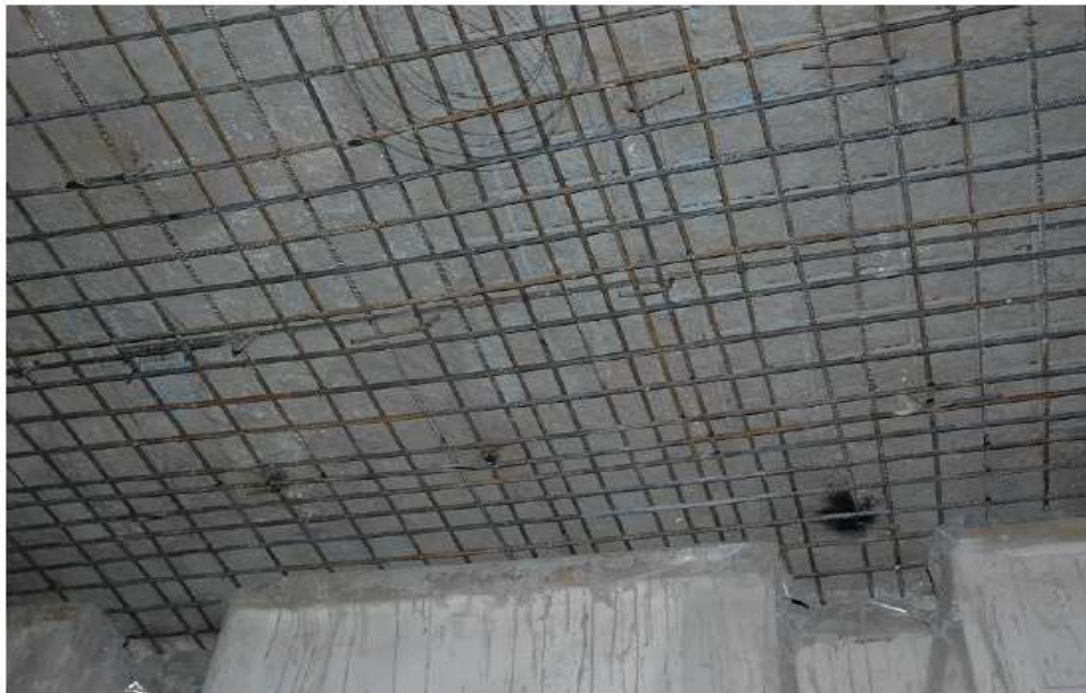
(e) Slab strengthening of the second floor
