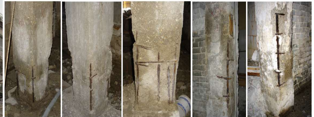
Figure 3: Corrosion of the steel reinforcement of the RC columns K17, K21, K24, K28 and K29 (ground floor)
