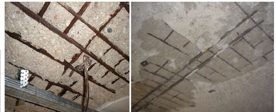
Figure 4: Extensive corrosion of the steel reinforcement of the RC slabs.
