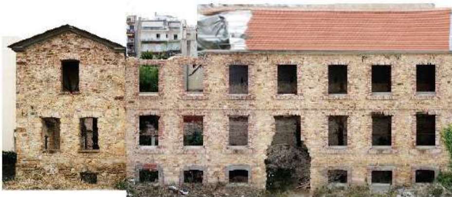
Figure 9. Rectified mosaic of images (left) and corresponding digitized façade (right)
