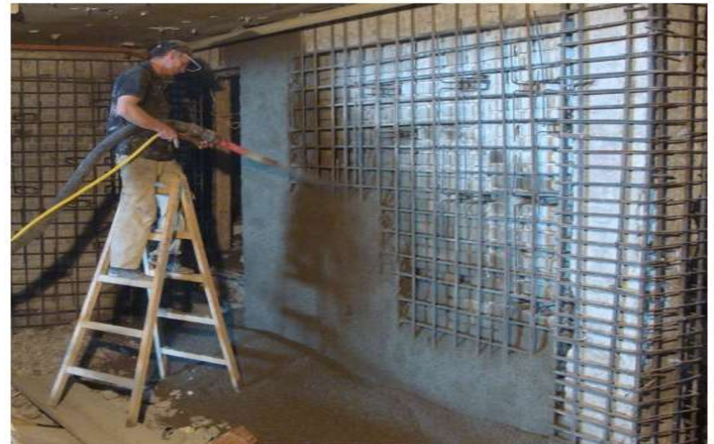
(f) Shotcrete application
