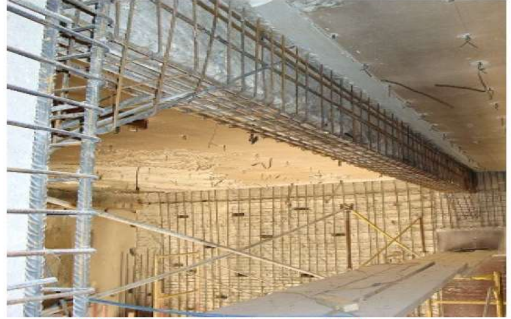
(d) U-jacketing of a beam with large span
