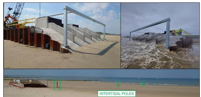
Figure 2. The artificial dike RDR and intertidal poles at low tide (top left and bottom) and high tide (top right).
