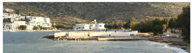
Figure 1. Katapola beach (2015) shortened by the pier consisted of embankment material and 17 concrete blocks.
