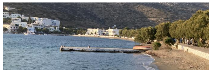
Figure 2. Katapola beach (2021) has been fully restored.
