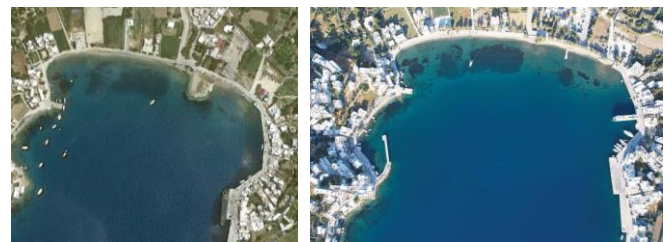
Figure 3 & 4. Satellite photos of Katapola bay before (3) and after (4) the construction of the fishing shelter (on the left).
