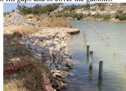
Photo 4. Banks' armor behind support columns. Works under construction!
